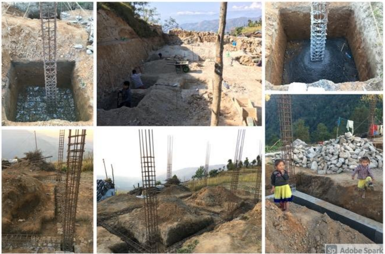
Foundations (top pictures) and footers (bottom pictures) of the new homes in Kholegaon. All construction was completed to the National Reconstruction Authority requirements to receive aid stipends.
