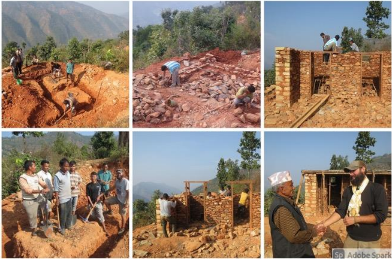
Patelshor Primary School sanitation system construction project 2015.
